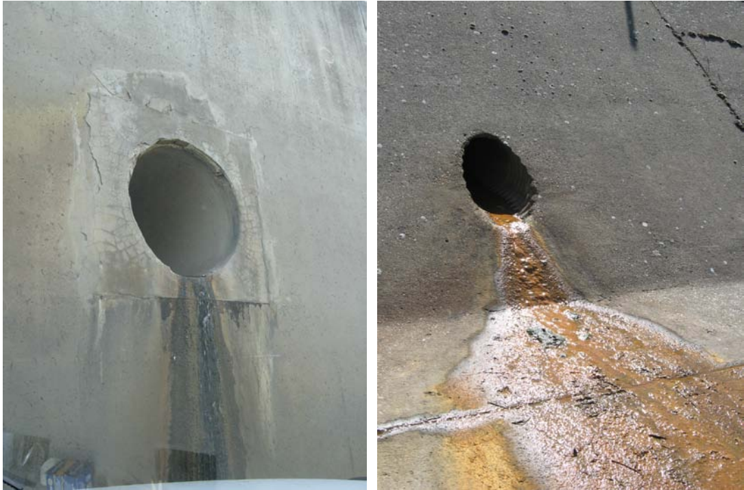
Figure 2: Typical outfalls in floodworks.
