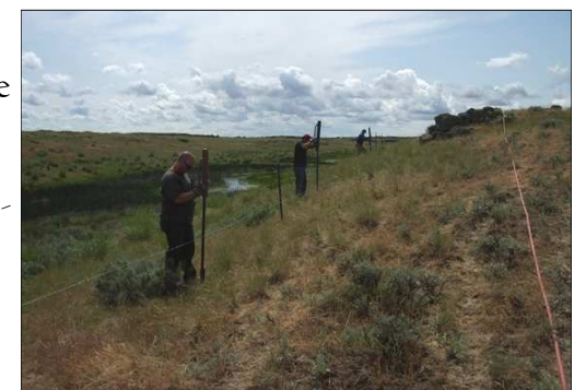
Conservation crew installing riparian fencing
