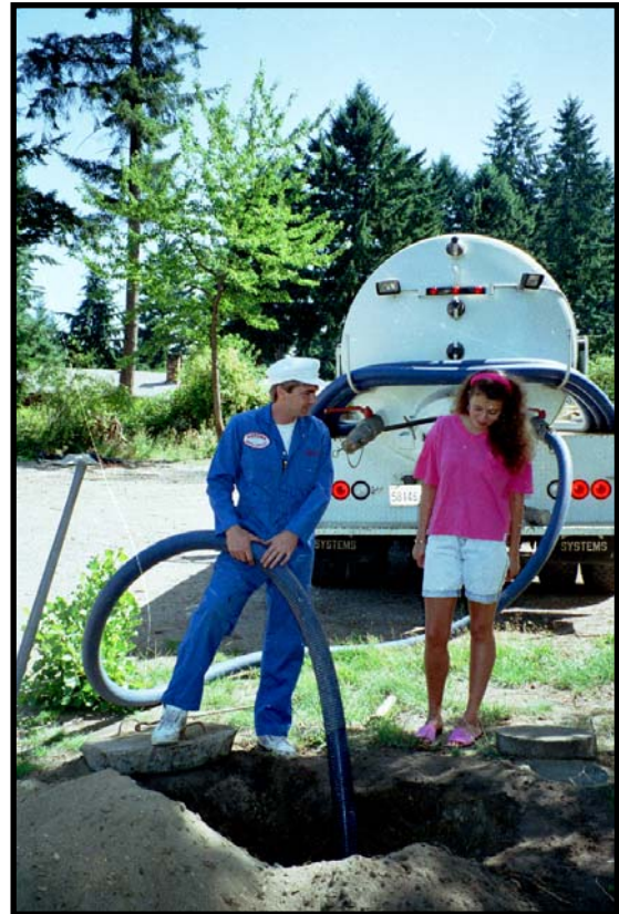
Figure 8. On site septic systems. Septic systems require servicing. If you have a septic system and the ground above it is wet, squishy, or smells bad, you should have it inspected and pumped as shown here.
