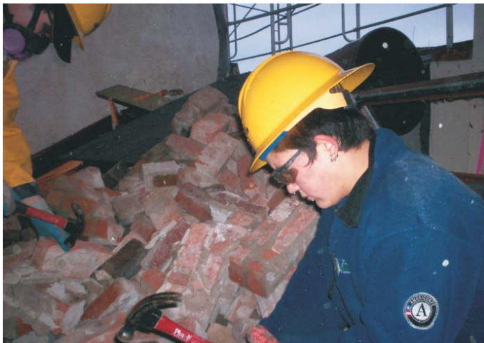
Sammy Harvell cleans mortar from bricks so that they can be reused
