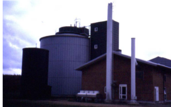
Figure 8: Grindsted, Denmark (Krüger Biosolid System)
