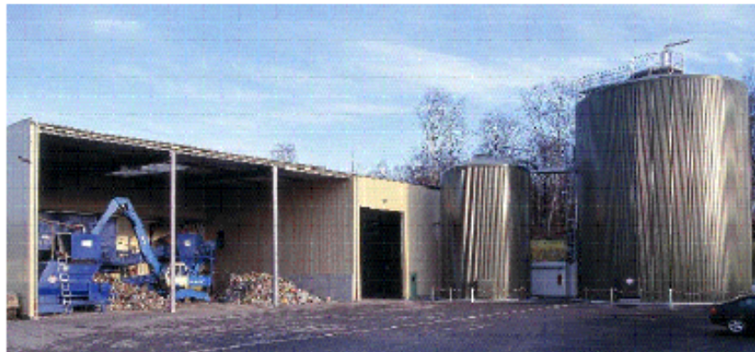
Figure 27: ISKA Dry Two-Stage Two-Phase system at Buchen, Germany
