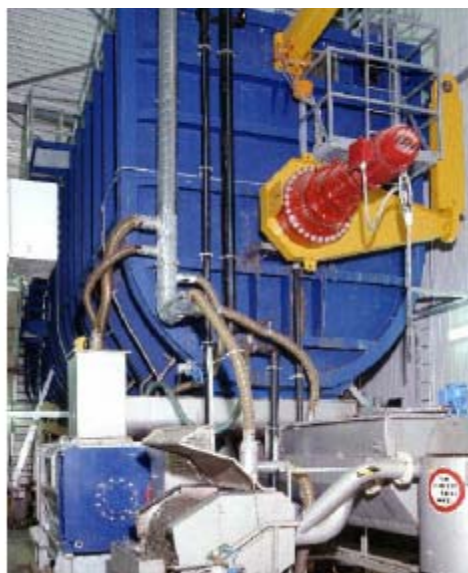
Figure 28 The first stage of percolation at Buchen, Germany
