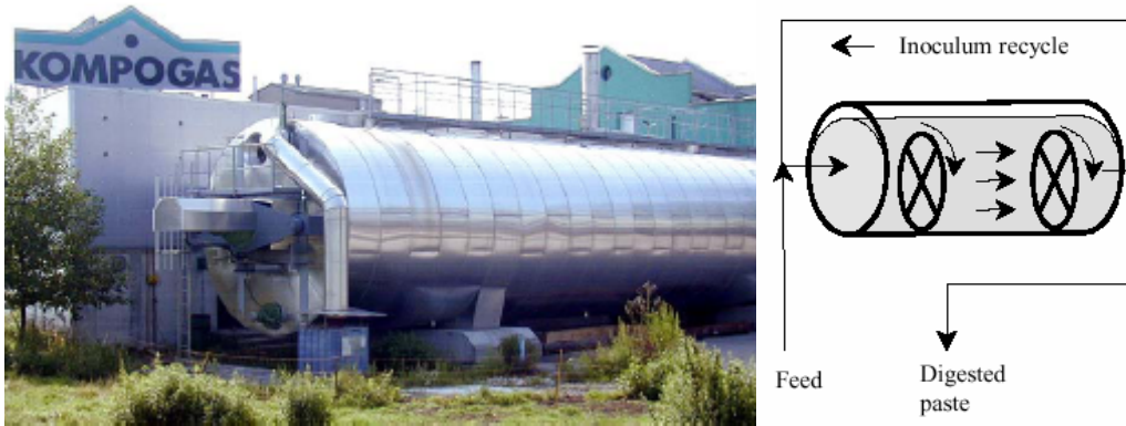
Figure 11: Installation at Niederuzwil, Switzerland, Kompogas system
