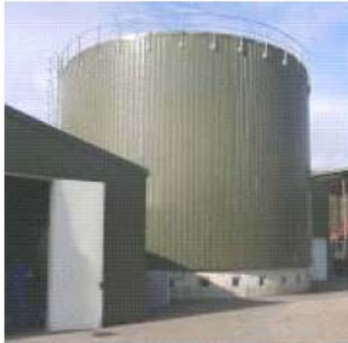
Figure 18: Valorga system installation at Geneva, Switzerland
