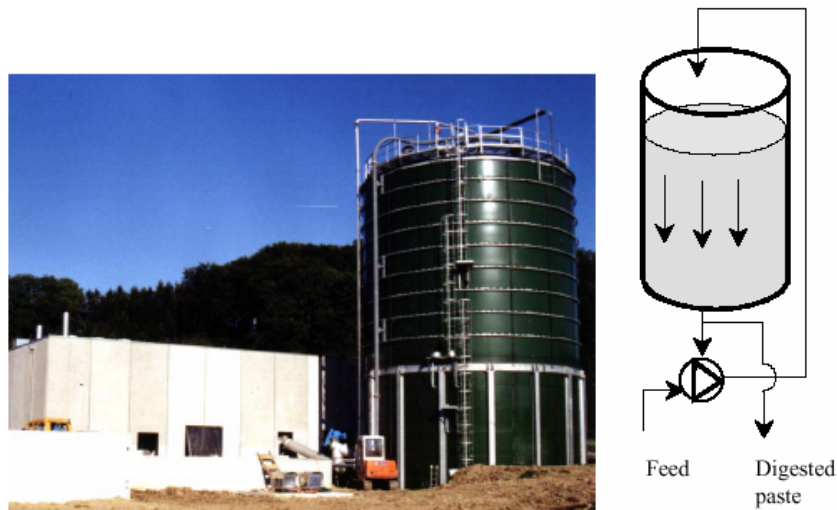
Figure 17: Dranco Solids Digester Installation at Aarburg, Switzerland
