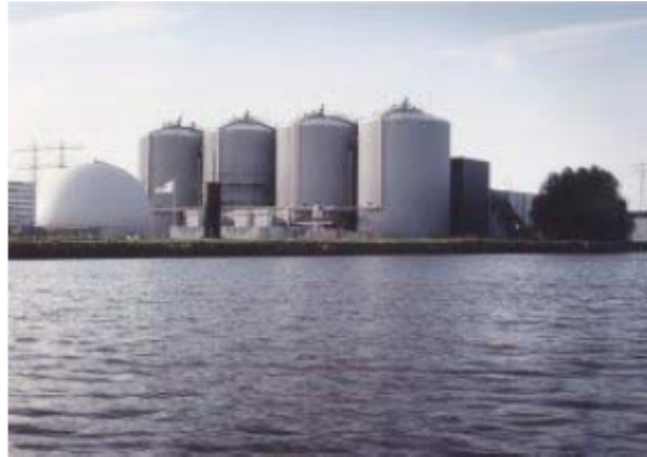
Figure 5 Vagron Wet Single-Stage digestion facility
