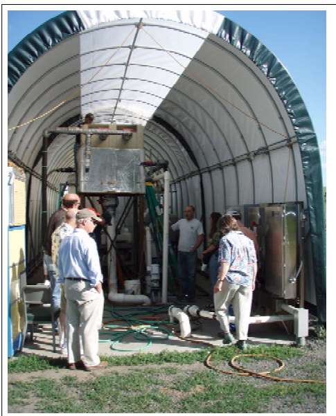
Washington State University’s anaerobic digester.
