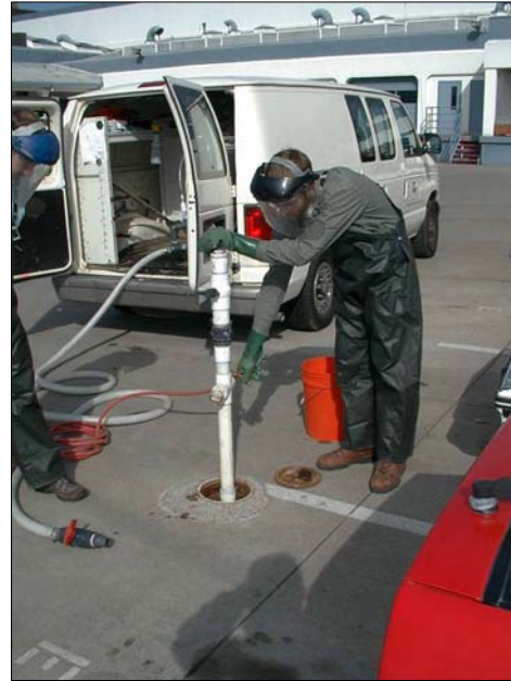
Cleanup using bioremediation with hydrogen peroxide injection at North yard. March 2001.
