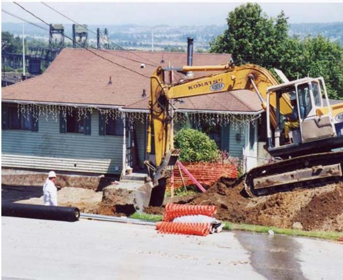
This is a picture of soil excavation. The contaminated soil will be placed into containers to be hauled off by truck from the site. The contaminated dirt will be disposed at a landfill approved to accept this contaminated soil.
