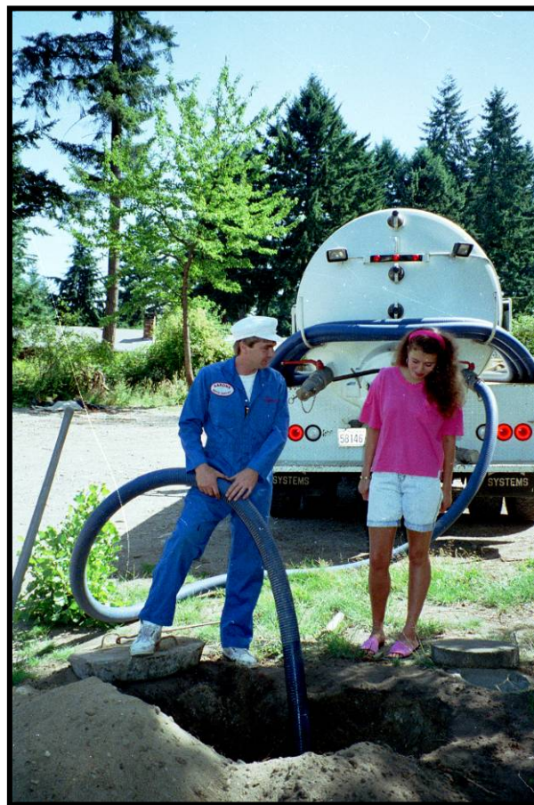
Figure 9. Onsite septic system care. If the ground above your septic system is wet, squishy, or smells bad, you should have it inspected and pumped as shown here.
