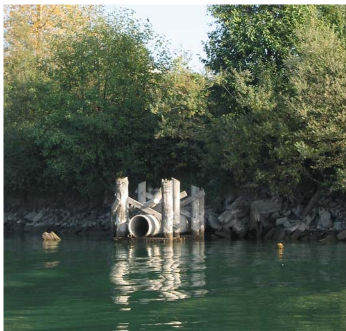
Figure 13. Park Street Combined sewer overflow outfall, Skagit River, Mount Vernon (photo: Dave Garland)
