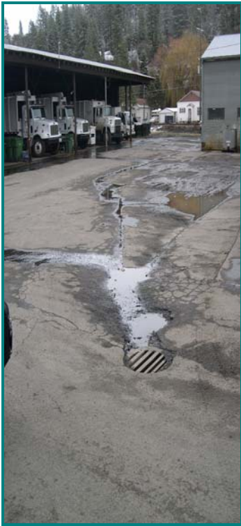
Empire Disposal's direct discharge to river
