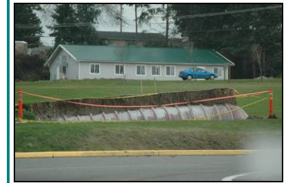
Freeland Plaza surge tank
