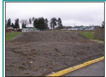
Surge tank in elevated mound
