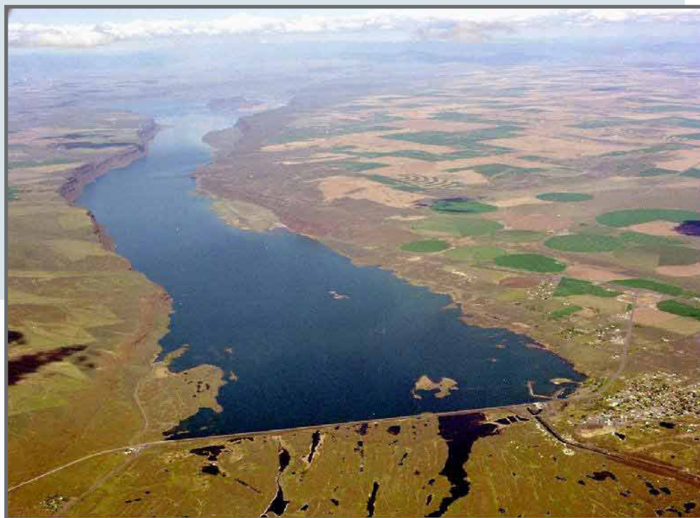
Dry Falls Dam on Banks Lake (source: USBR website)
