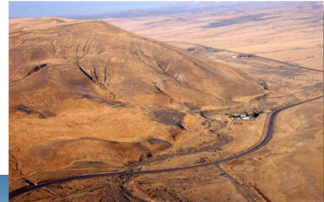
Dave Walsh, USBR: Aerial view of Black Rock damsite, looking west
