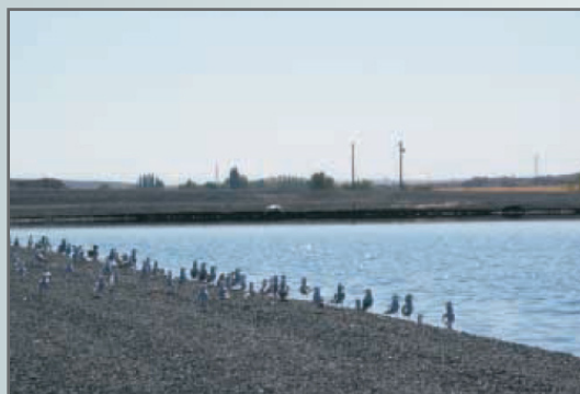
Ephrata groundwater recharge basin
