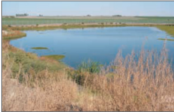
Royal City's infiltration basins.
