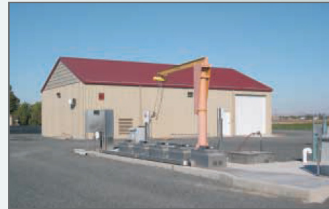
Quincy's treatment & control building with UV channel in front.
