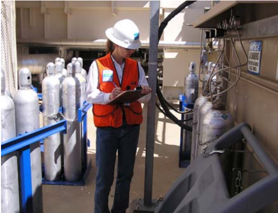
Lynnette Haller, air quality engineer, inspecting calibration gas canisters for a continuous emissions monitoring system.
