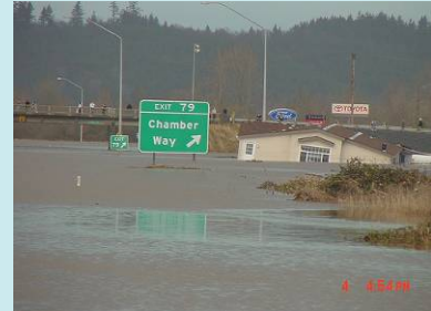
I-5 at Chamber Way exit in Centralia
