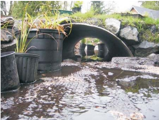
To slow the flow of water down, these sedges will be planted in a "half moon" fashion alternating along the rain garden
