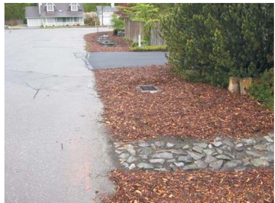
The rock pathway was innovatively designed to suit both homeowner and stormwater needs
