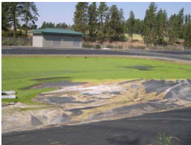
Liner under the lagoon
