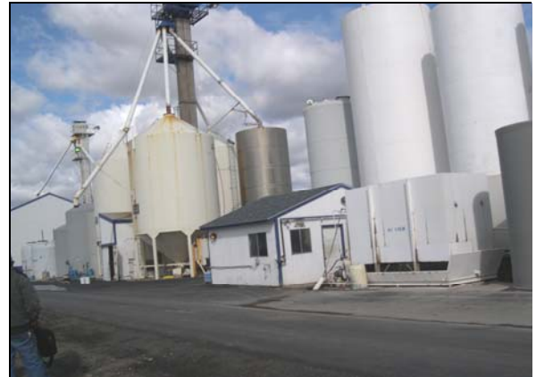
NU CHEM's Central Ferry Facility
