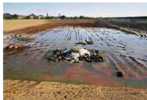
Initial deliveries to the project, January 2, 2003 (Basin 2B)
