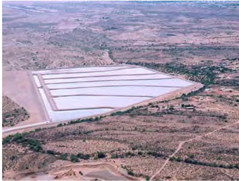
Recharge Operations at Constructed Facility
