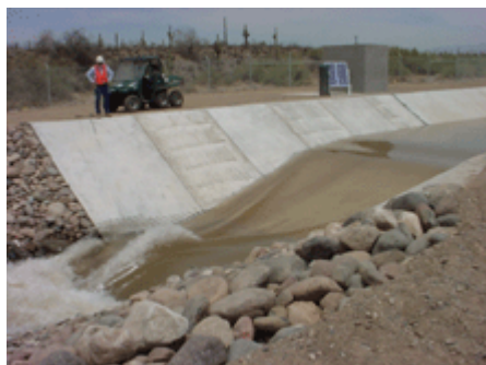
Broad-crested Weir above Recharge Basins
