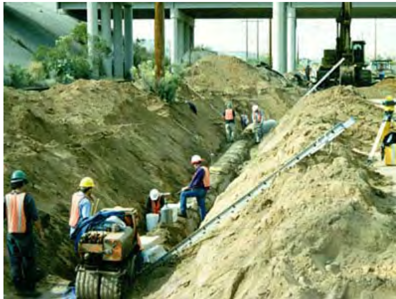
Placement of Delivery Pipeline Under the I-10 Freeway
