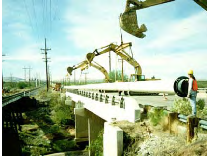
Construction of the Isolation Valve Vault and Flowmeter Vault
