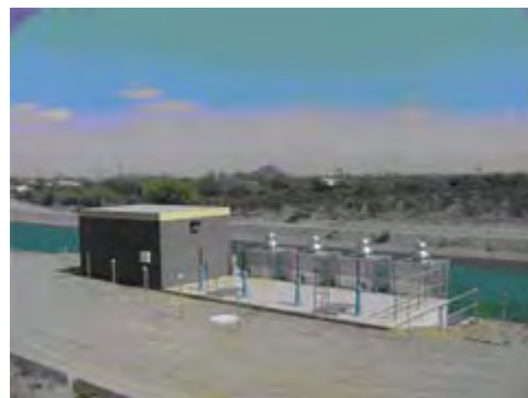
Pump station at HMRP
