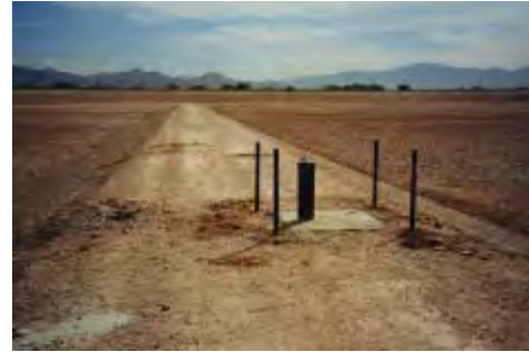
Piezometer PZ-3 Located Between Basin 1 and Basin 2
