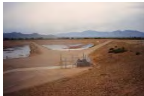
High Infiltration Rates Have Allowed Basin Rotation to be an Effective Tool for Controlling Algae
