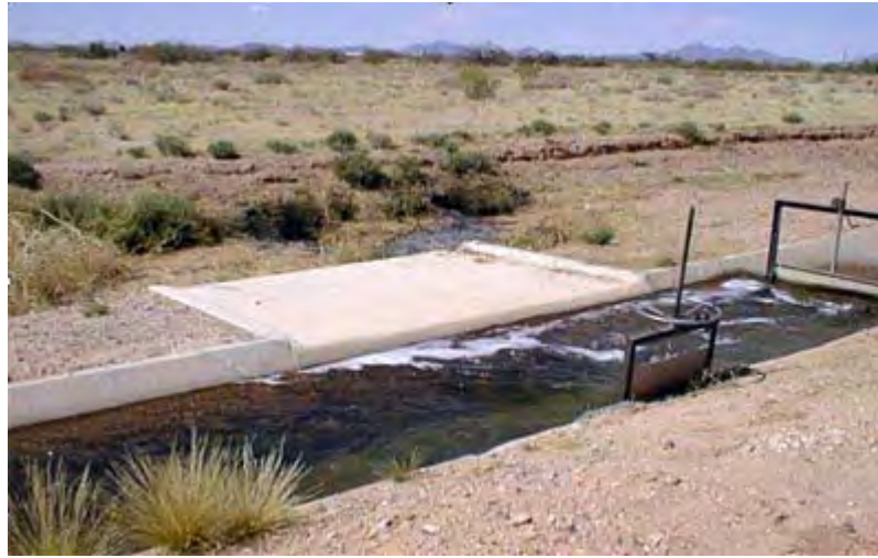
Manual slide gate to divert water into recharge project
