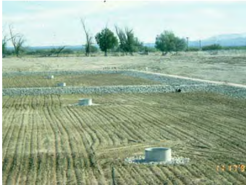
Basins Excavated and Ready for Recharge
