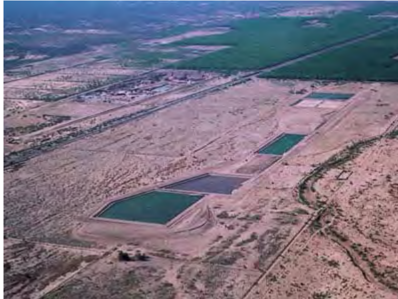
Operation of Three New Expansion Basins Down Slope from the Original Pilot Basin
