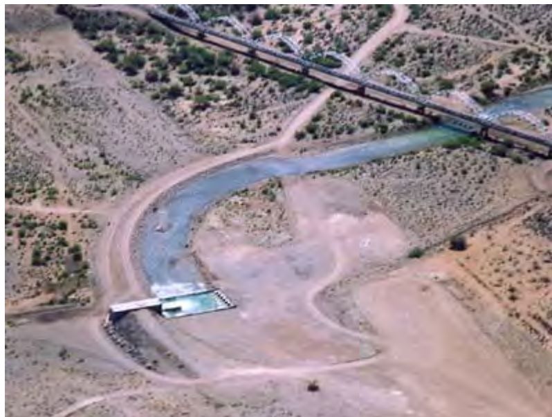
Release into Agua Fria River via Blowoff Structure
