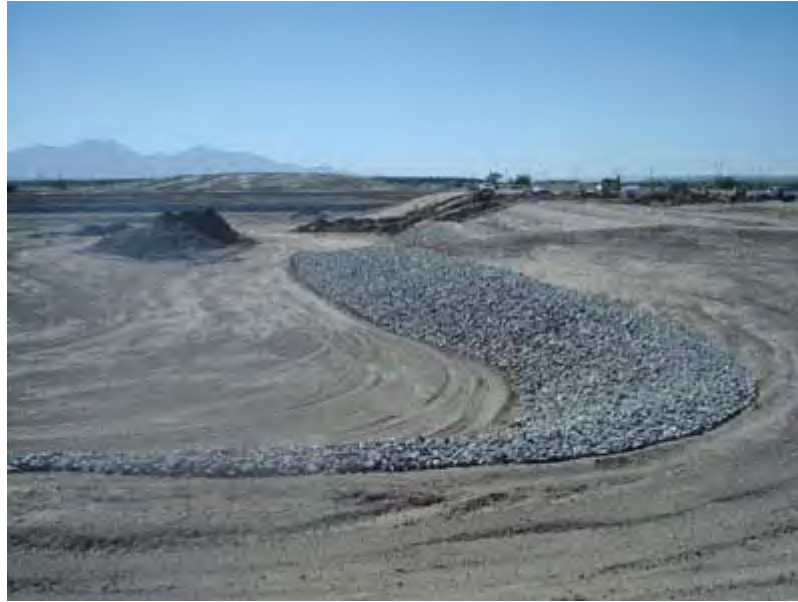
Construction of Basin 3
