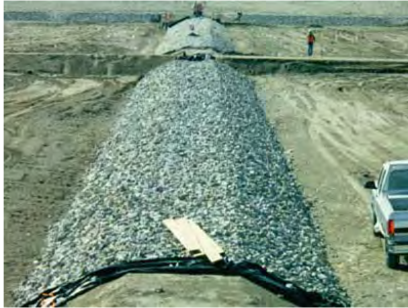
Rip-Rap Placement on Divider Berm
