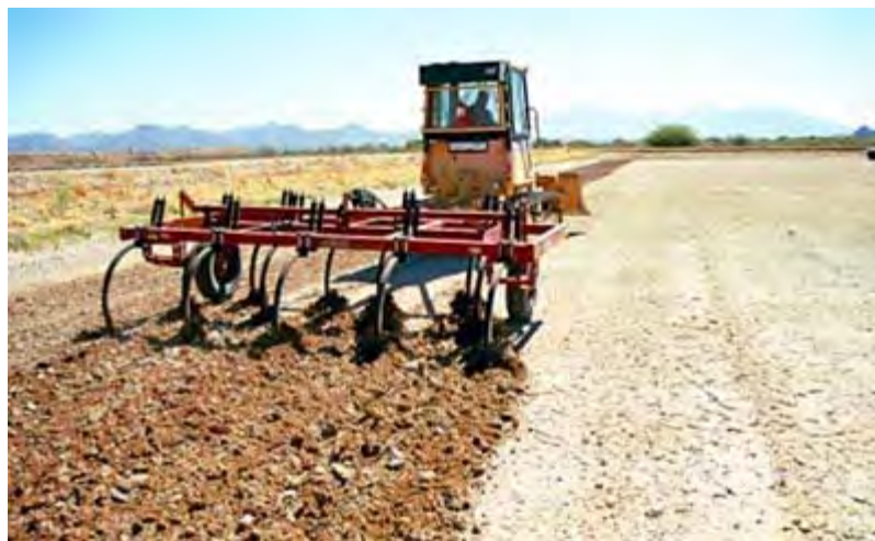
Ripping the basin bottom using the spring-toothed harrow.
