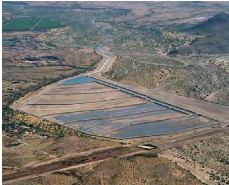
Water Captured from River at Headworks Structure for Delivery to Recharge Basins
