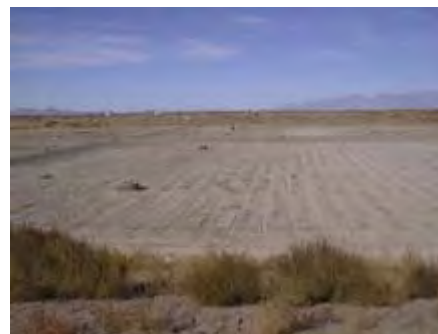
View of Pilot Basin After 40,000 AF Recharged. Notice Hard Encrusted Surface Layer that Reduces Infiltration Rates.
