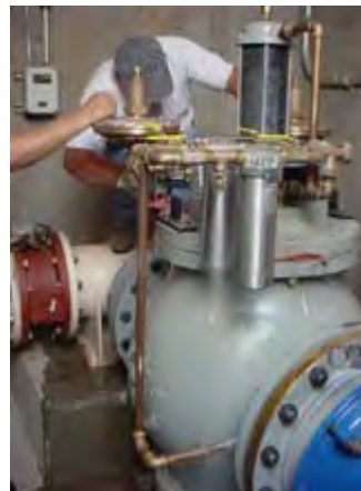
Maintenance Crew Fine Tunes PRV Valves That Were Installed in July 2003
