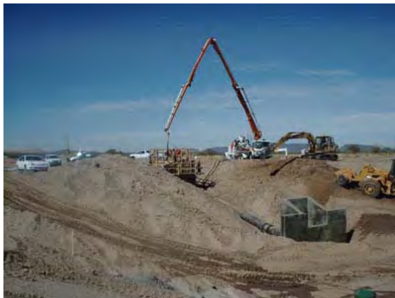
Construction of a Basin Turnout
