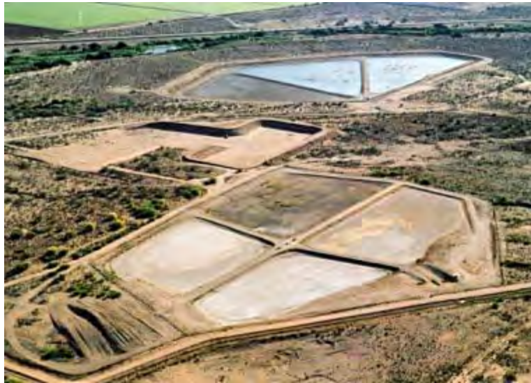
Aerial view showing the proximity of AVRP in the foreground and LSCR in the background
