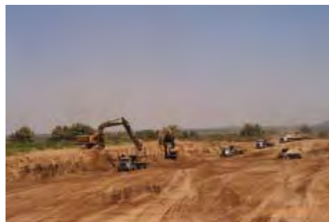
LSCR Basins Being Excavated During Construction
