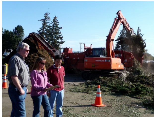
Gary Bleeker (left) and Canming Xiao (right) discuss operations at the Kittitas County Compost Facility with Patti Johnson (center), Kittitas County Solid Waste Director. The facility was built using Coordinated Prevention Grant funds to provide a recycling alternative to burning or landfilling yardwaste.
