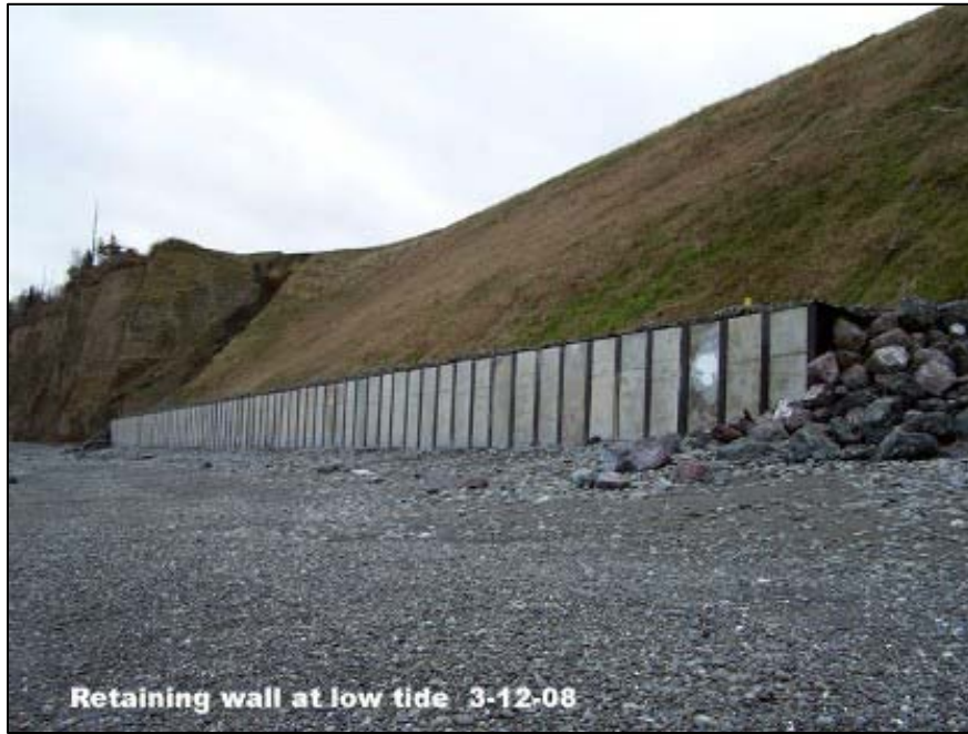
Figure 3. Stabilized Slope and Seawall at Base of the Closed Landfill, March 2008.
