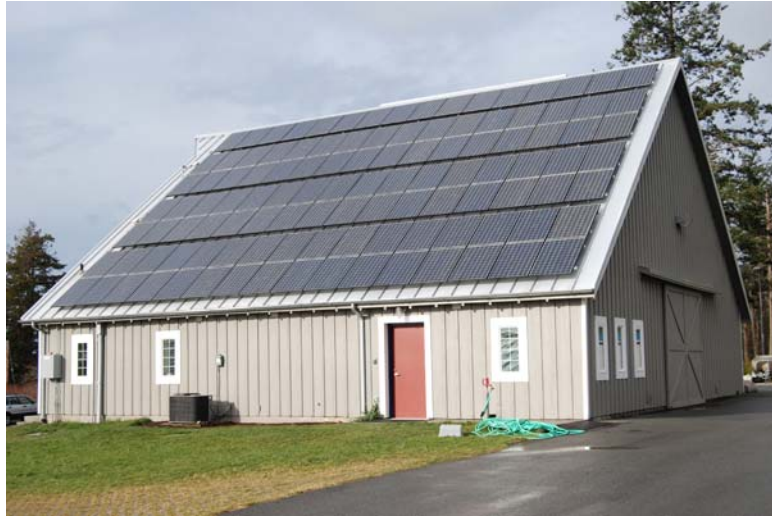
Photovoltaic solar generation system on the barn roof
