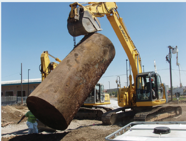
Figure 3. Removal of an underground storage tank which contained oil with PCB contaminants.
