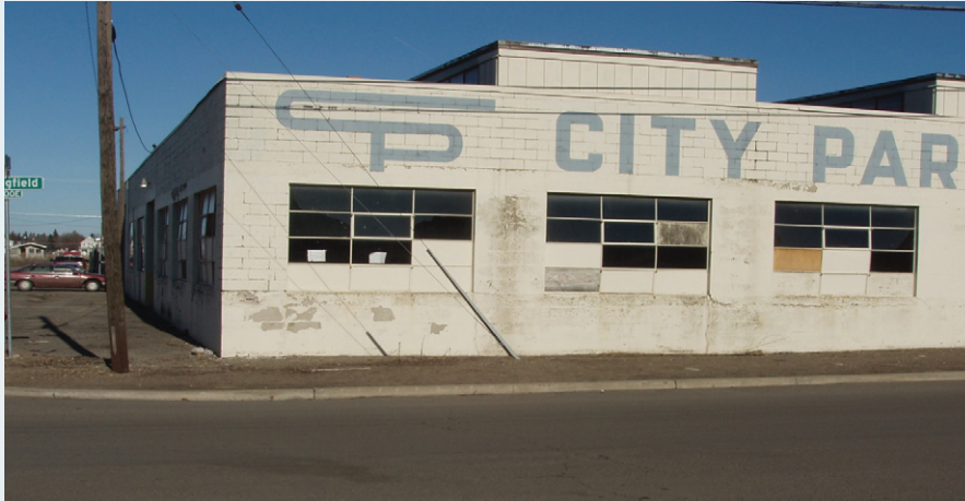
Figure 1. This is the City Parcel property with the building still standing before the cleanup actions began.
