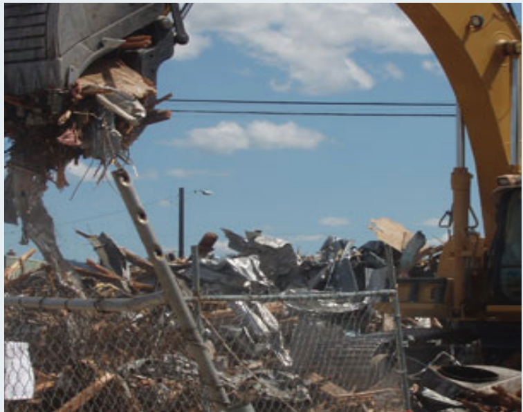
Figure 2. The City Parcel building was demolished to clear the area for the removal of the drain lines, dry wells, and underground storage tanks, and to access the soils for systematic excavation.
