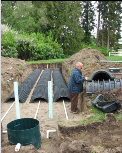
Installation of gravel-less dome chamber system
