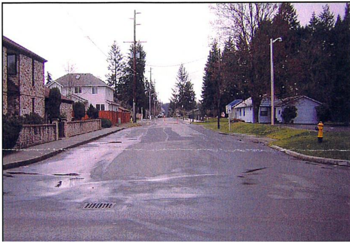
Decatur Street before construction. By Craig Tosomeen
