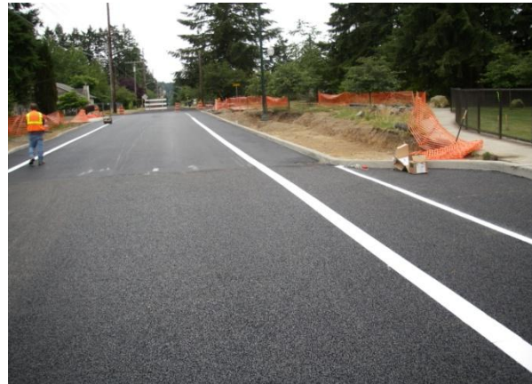
Pervious to impervious pavement. Rain gardens on the side will treat runoff from impervious pavement. By Craig Tosomeen.
