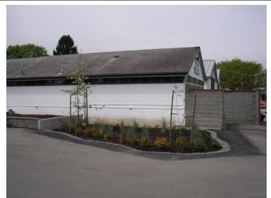
Rain garden installed to infiltrate runoff from adjacent road and building roof.
