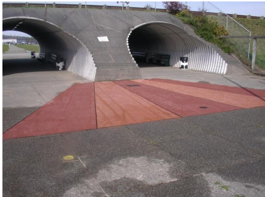
Two types of porous concrete installed at the fairgrounds entrance.
