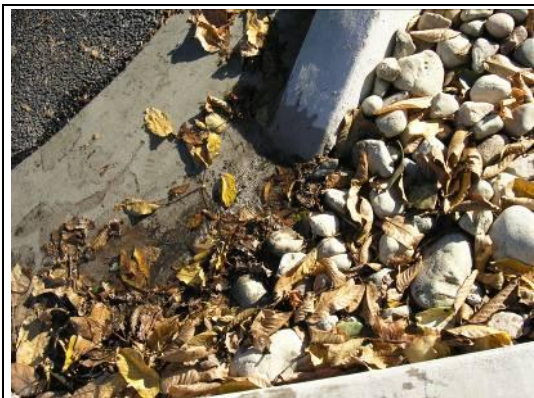
Leaf litter alongside the rain garden could be a small maintenance issue.
