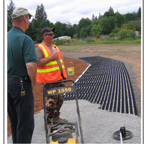
Installation of Gravelpave2.
