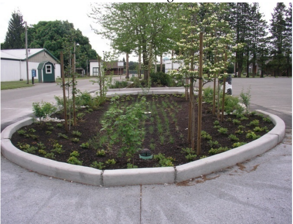
Local stormwater management with LID
