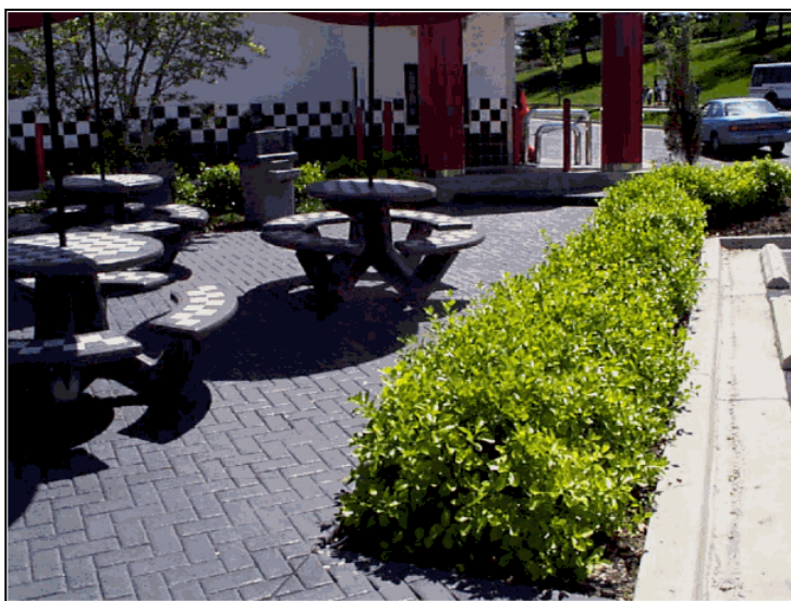
A stormwater-friendly hard surface.
