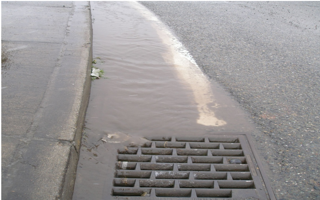
Figure 7. Stormwater Pollution. Stormwater can carry a variety of pollutants including sediment, household products, metals, fertilizers, bacteria, and phosphorus. Some of these pollutants enter Rock and Ravensdale Creeks and eventually enter Lake Sawyer.
