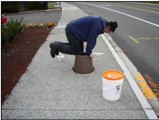
Testing infiltration of permeable concrete.
