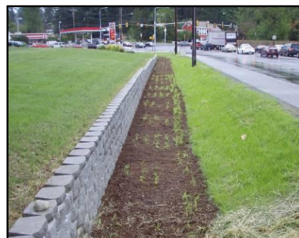
View of linear bioretention feature and permeable concrete sidewalk along Military Road South.
