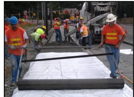
Pervious concrete sidewalk installation.
