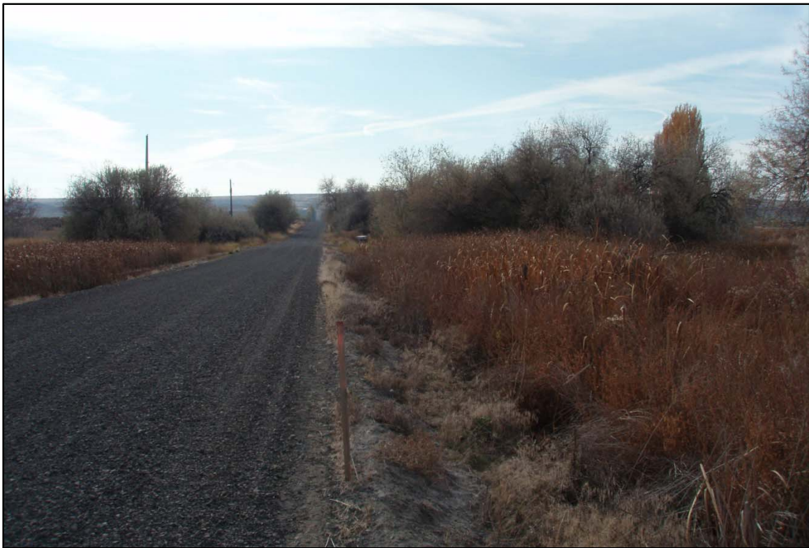
Figure 6. South facing view of the project area, note raised road prism and riparian vegetation.
