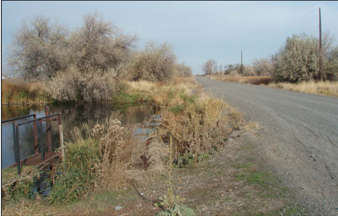
Figure 5. North facing project area view, note road prism above Wasteway pipes.
