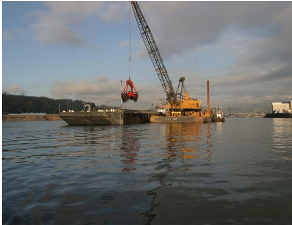
Dredging in the Duwamish River with the West Seattle Bridge in the background.
