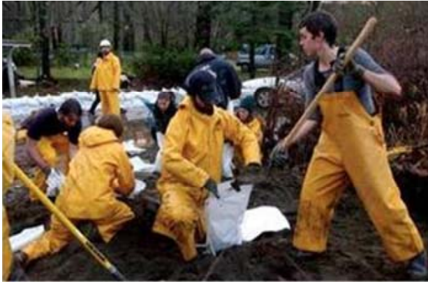
A Washington Conservation Corps crew (clad in yellow rain gear) led by Troy Warnick (white hat) frantically fill and stack sandbags in an effort to prevent flooding in the Nisqually Valley. Crewmembers from left to right include Jason Smith, Ben Amidon, Wade Arnold, Courtney Irby, and Ana Hansa-Ogren (with shovel).
