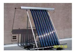
*Photo 4: A Solar thermal water heating system installed by staff at Yakima Valley College.*
