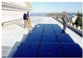
Photo 11: GA installed solar panels with the help of Puget Sound Energy. GA uses the panels to power the lights at the top of the dome of the
