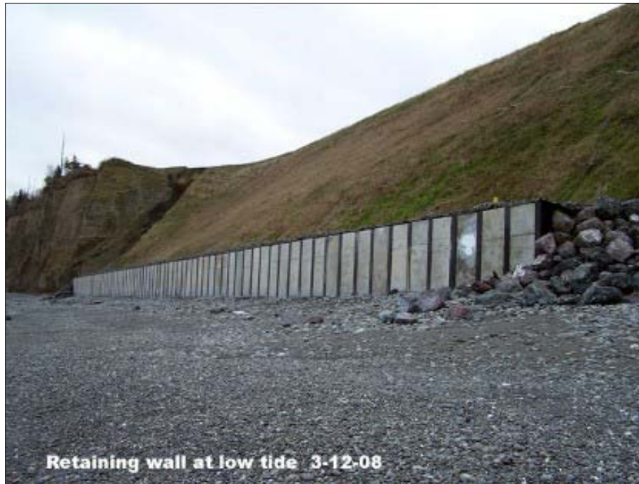
Figure 3. Stabilized Slope and Seawall at Base of the Closed Landfill. Photograph by Dry Creek Coalition.
