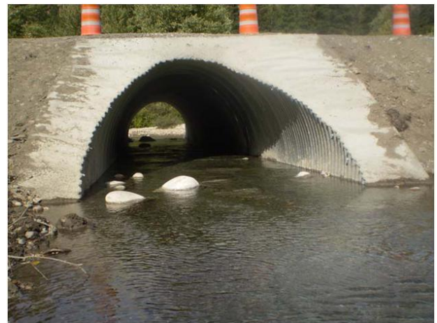
Figure 2. Outlet of oxbow after reconnection.
