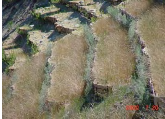
Use of biosolids in slope stabilization along U.S. Highway 97A in Chelan County (background, no biosolids; foreground, biosolids compost)
