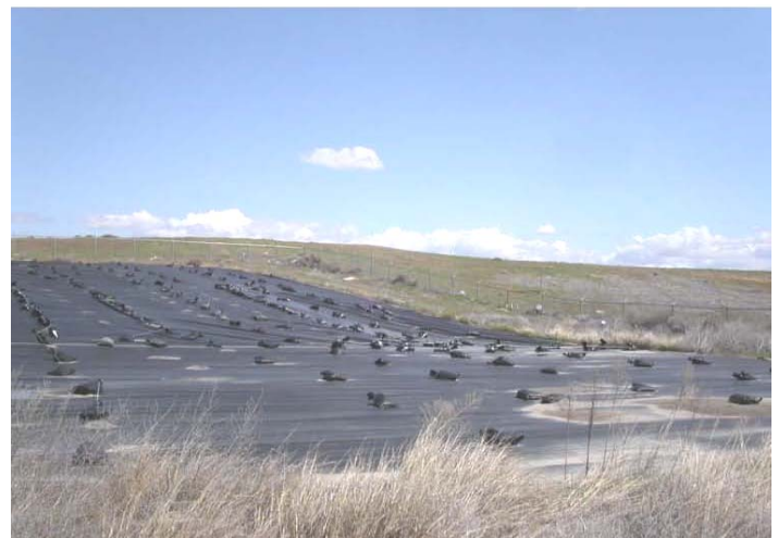
Photo Courtesy of AMEC Current Temporary Landfill Cover for Zone B
