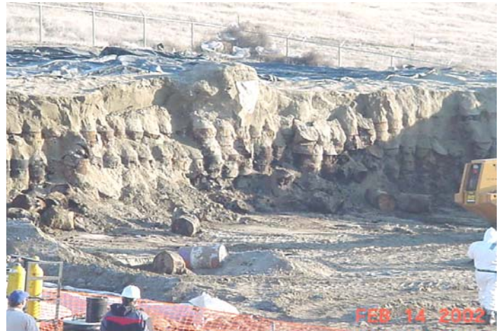
Removal of Zone B Drums
