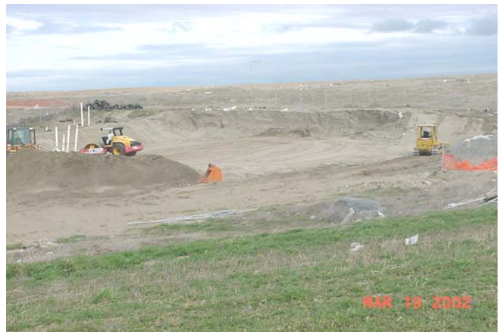
After Zone B Drum Removal
