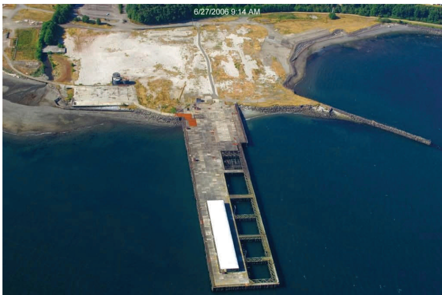
Aerial view of the Rayonier Mill property and dock
