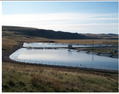
Lined wastewater ponds
