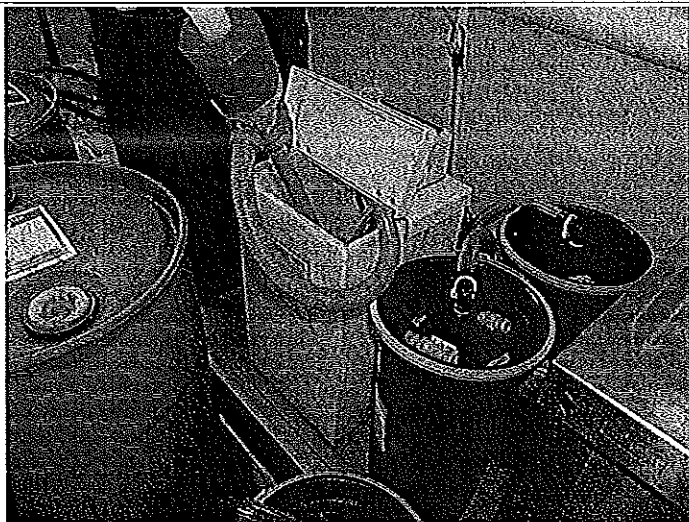
PHOTO #:27 DATE: JULY 19, 2009 TAKEN BY: AMY JANKOWIAK FILE No.: P7190050 DESCRIPTION: PHOTO SILVER RECOVERY SYSTEM
