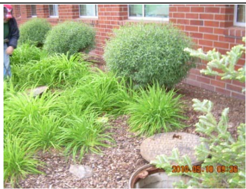
Rec Center Grease Interceptor to reduce the amount of grease and oils that reach Cheney's treatment wastewater plant.
