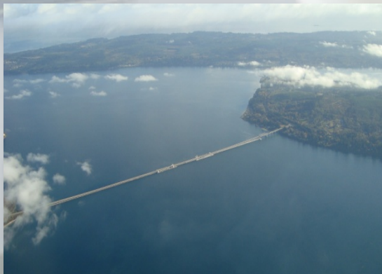
Hood Canal Bridge
