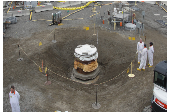
Area prepped for removal of C-107 riser.
