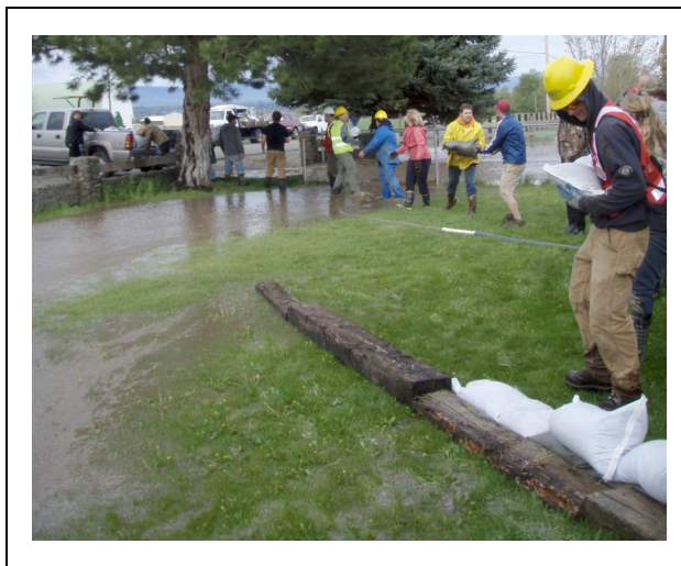
Yakima Crew member Trinity Peterson receives sand bags from a fire line of volunteers and places them in the barrier
