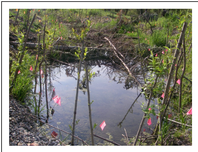
Budding willow stakes on the stream bank at South Silver Springs
