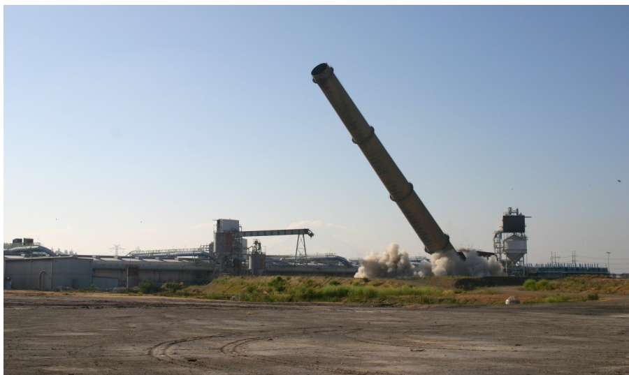
Former Kaiser Aluminum Company plant demolition
