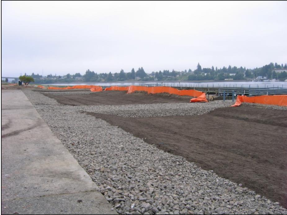
**Figure 31. City of Bremerton Parks Dept LID retrofit project at Lions Park:** *Biofiltration cells will capture and treat stormwater that previously discharged to Port Washington Narrows.*
