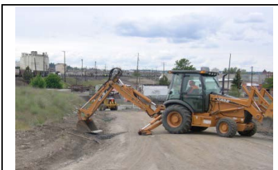
Construction of rock flow control structures
