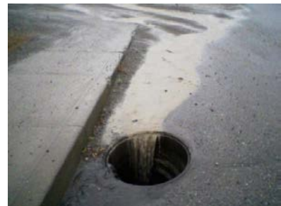
Turbid stormwater running into storm drain on Madelia Street
