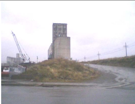
Stormwater running off BNSF's dirt access road to Madelia Street
