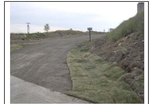
Newly sod-lined ditches to slow and filter runoff
