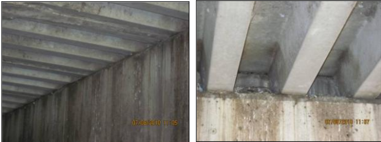
Figure 9. Underside of bridges over Spring Flat Creek in Colfax, WA. Note pigeon droppings on side of wall.
