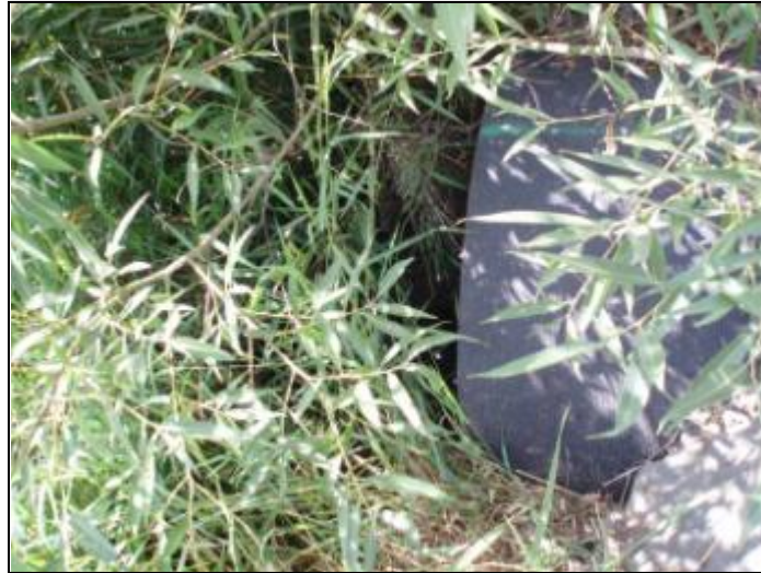
Figure 8. Example of a stormwater outfall that had consistent high bacteria concentrations (SFPRWSU1)
